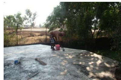
Painting lime to roof of animal house.
